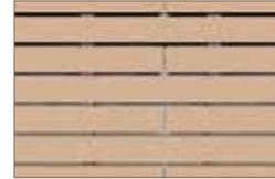
We recommend the formation of staggered joints (ship's deck pattern). In this case the lining-up of the joints can be accomplished more neatly and the mounting tolerances are less visible.
