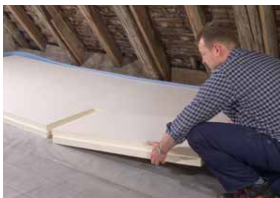
Insulation an attic floor with LINITHERM PGV
